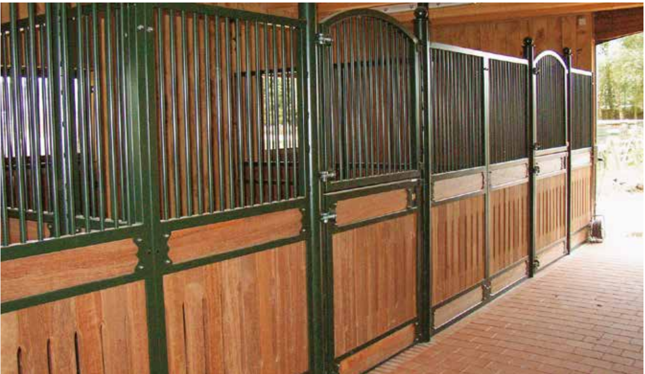
Image below: Belamie front wall with Ekki wooden panelling, powder-coated in addition
